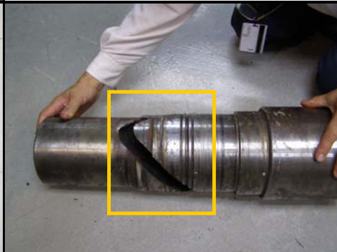
Turbine Shaft Failure
